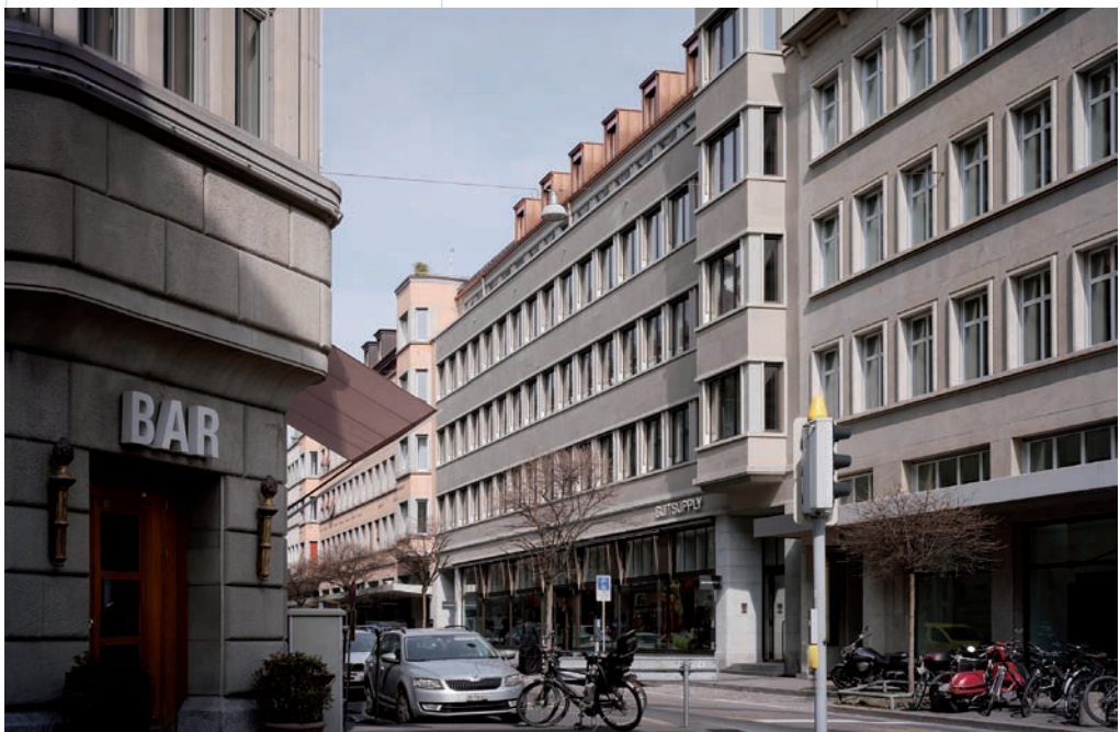
Nüschelerstrasse 24, Zurich, refurb project, to be completed in 2015
