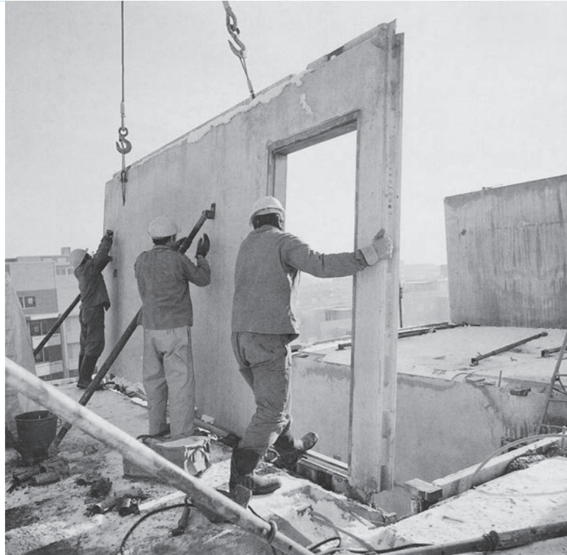
Göhner building constructed using prefab elements in Volketswil, in 1966
