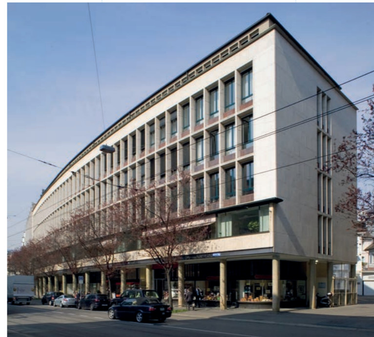
Bleicherhof commercial building, Zurich 2020
